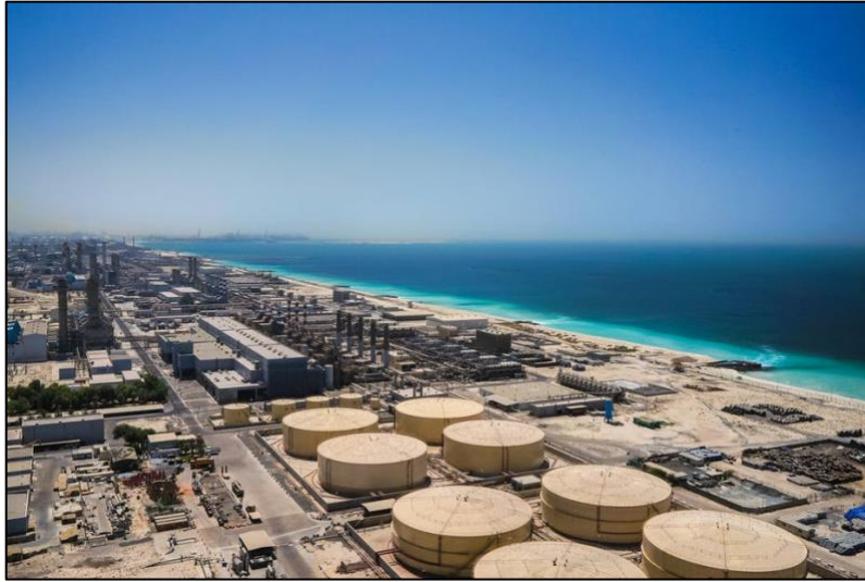
Figure 7 - Modern desalination plant, Arabian Gulf (Shutterstock)
