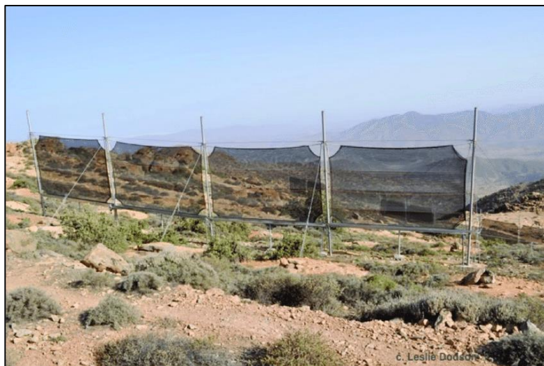
Figure 8 - Fogwater harvesting system in Morocco, includes 600 square meters of fog nets. (Photo by Leslie Dodson) - used under the Creative Commons Attribution-NonCommercial-NoDerivatives 4.0 International )
