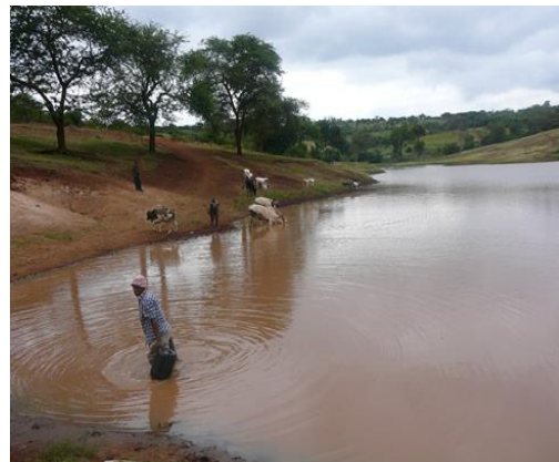
Figure 31: KKEDSHG dam not protected or fenced no water points hence contamination, photo by J. Mang'era
