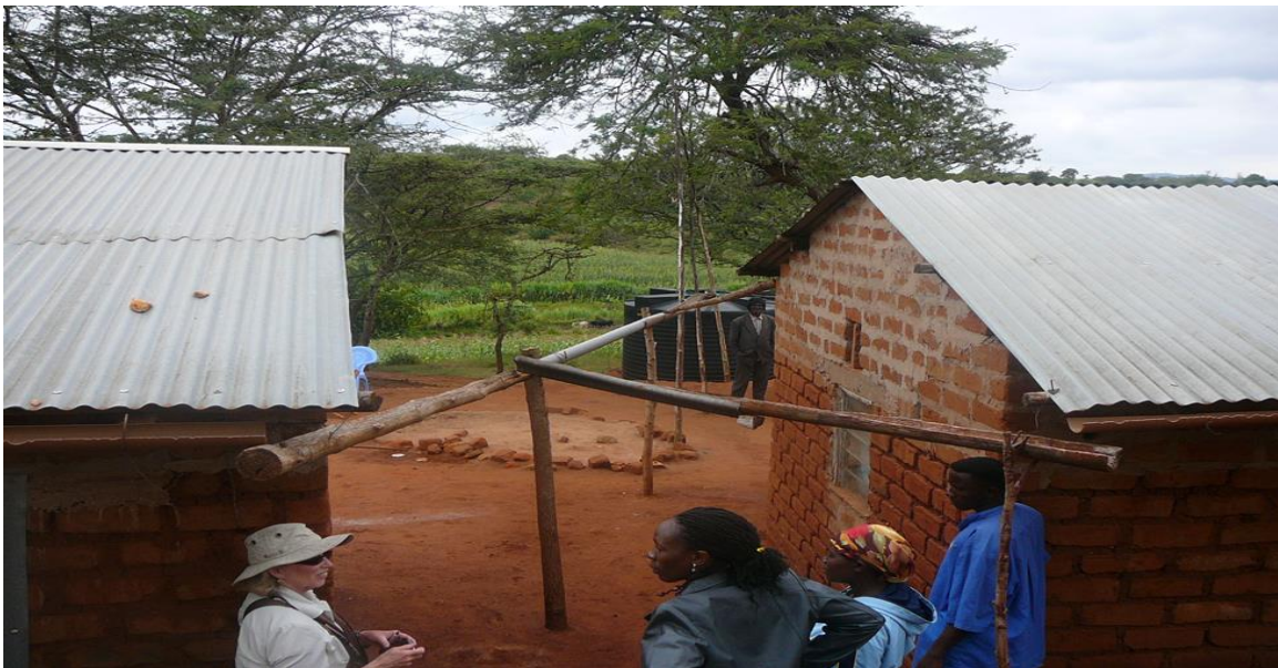
Figure 32: Improvised local materials in use for RWH. Photo by J. Mang'era
