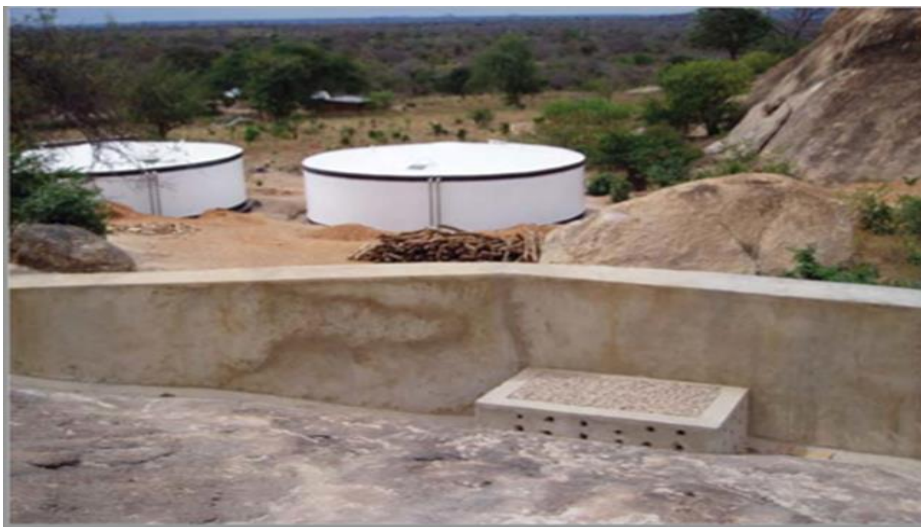
Figure 27: Muliluni Rock Catchment in Makueni County showing distribution tanks ( USAID/ Welt Hunger Hilfe,2009 )
