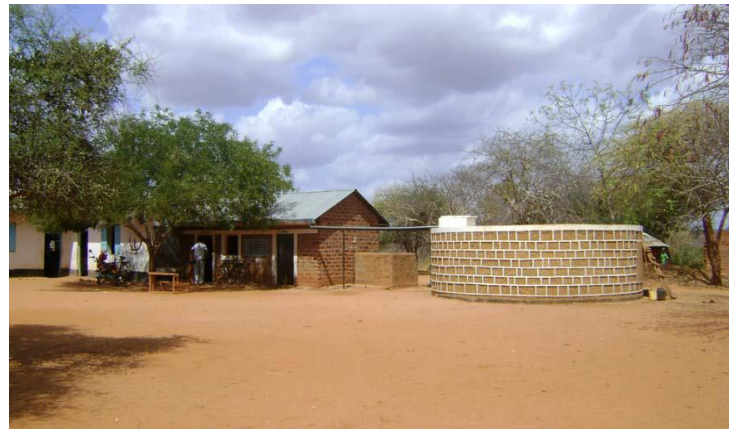
Figure 25 : Ferro-cement tank for roof catchment Source : Aroka (2010)
