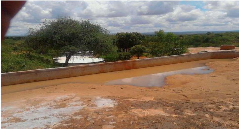
Figure 26: Rock catchment managed by Vololo self-help group with tanks together with distribution , Photo by J. Mang'era
