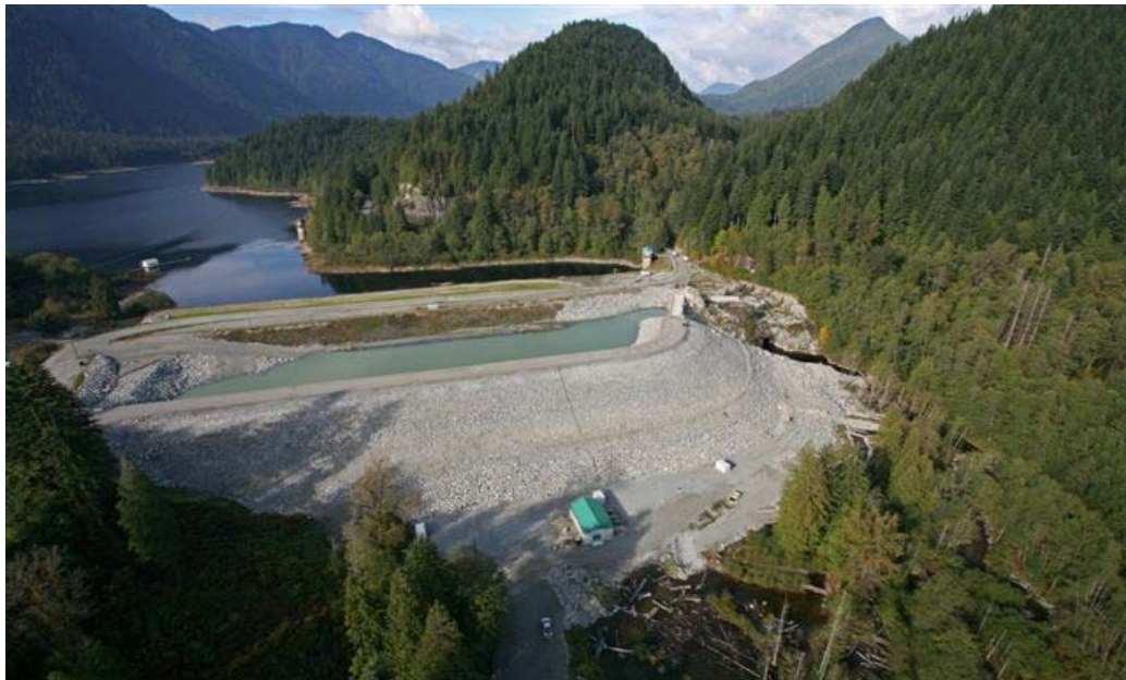
Figure 2: Photo of the Coquitlam Dam, Reservoir and CWSA (Source: BC Hydro, 2008).
